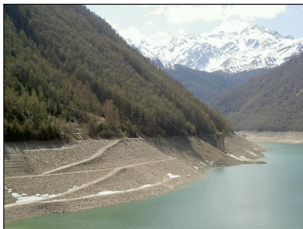
Fig. 8 – Southern slope – Stabilizing embankment
